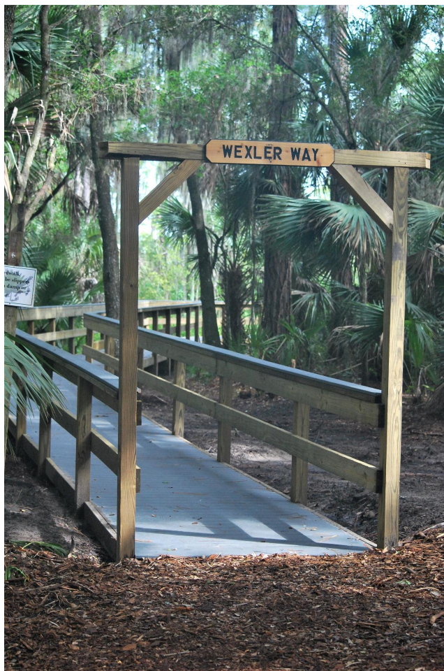
Entrance to renovated boardwalk
